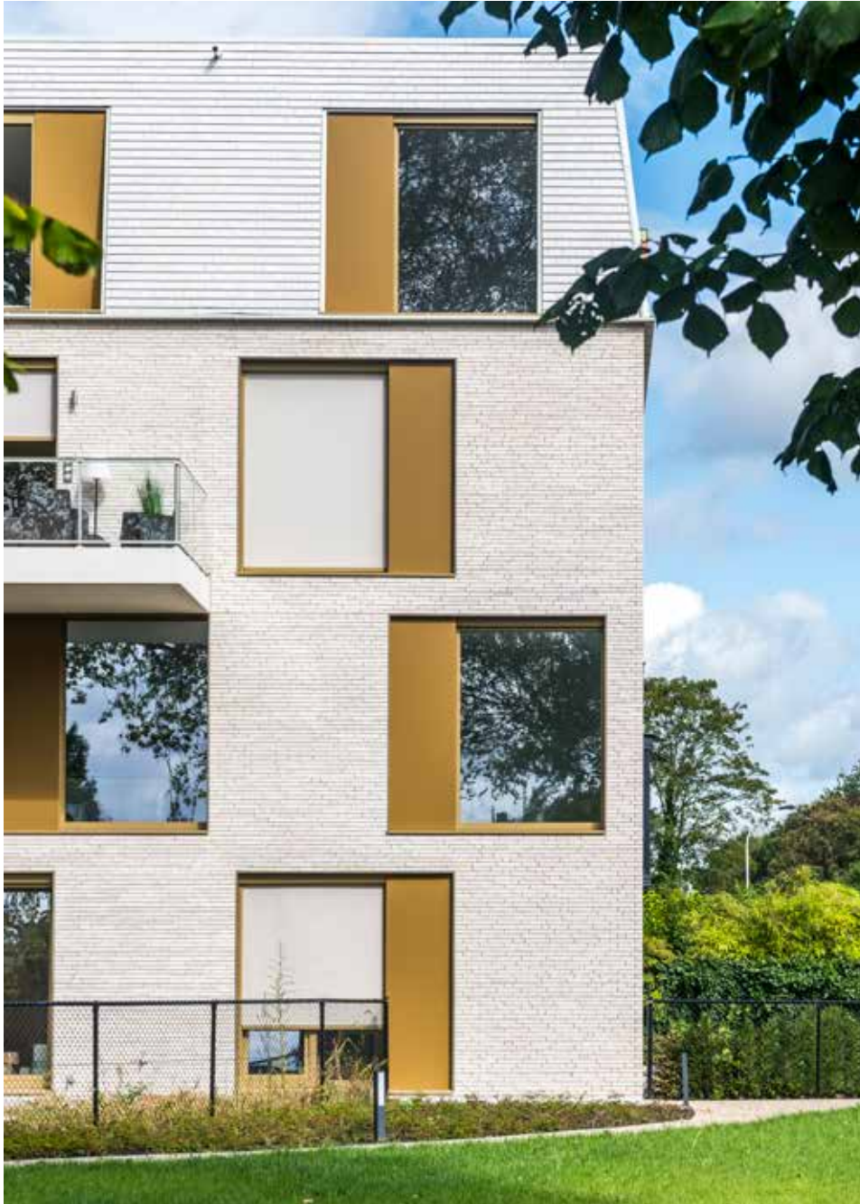
Façade: Terca Elignia Arctica White. Roof: Koramic Plain Tile 301 Cream-white glazed (special production)
