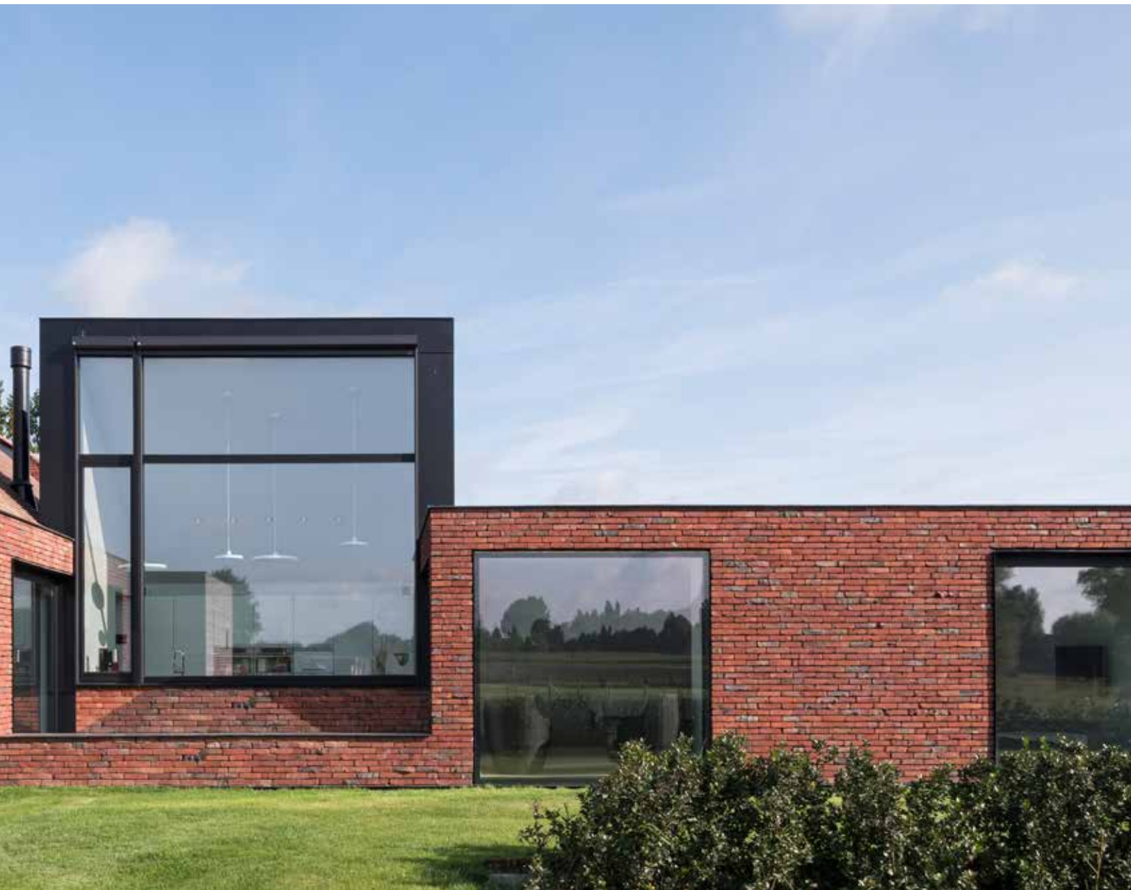
Façade: Brick-mix of Terca Artiza Hectic and Artiza Hectic Extra. Roof: Koramic Aleonard Esprit Patrimoine mix of Vineyard Black, Lichen Green and Kent Red
