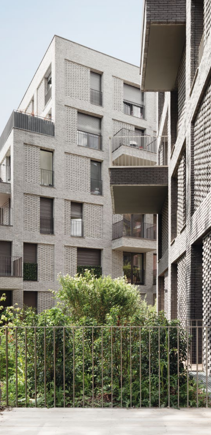
Left: The specific design of the façades and the laying of the individual bricks demanded the special expertise of craftsmen. Therefore, professional façade designers were engaged for this purpose.
