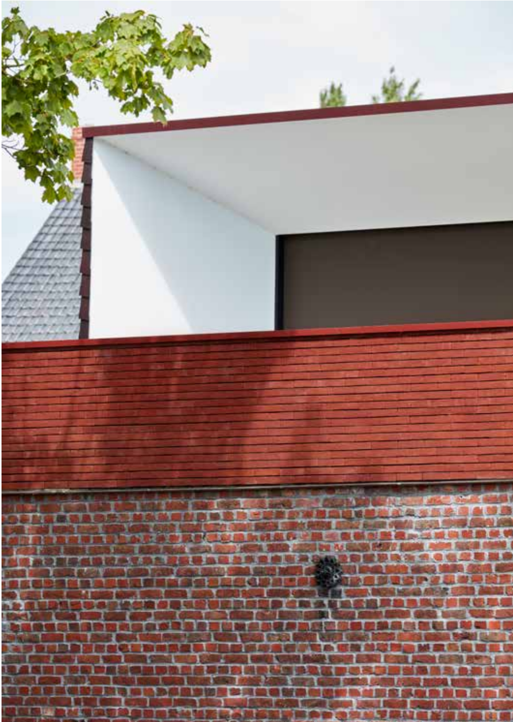
New volume and penthouse: Terca Egala Elise and Koramic Plain Tile 301 Wine Red Glazed
