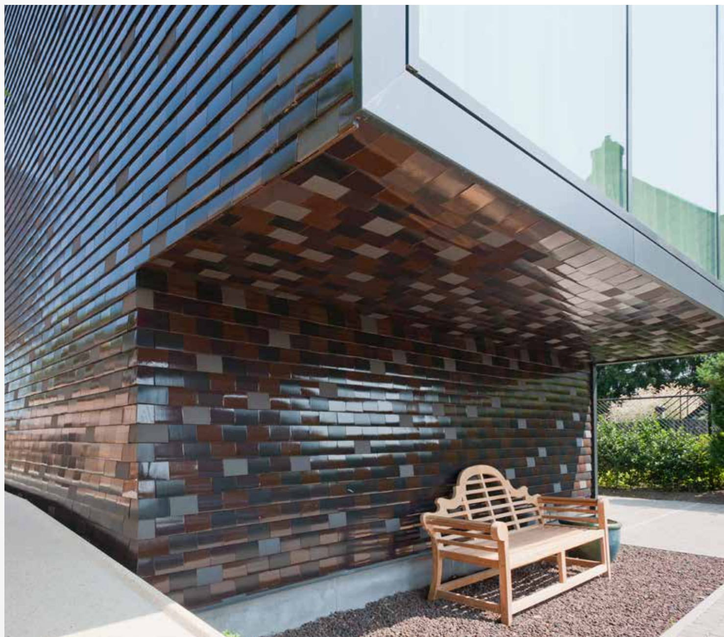
Koramic Plain Tile 301, mix of 28% Wine Red Glazed, 30% Brown Glazed, 10% Braised Blue and 32% Anthracite aNNo Architecten, Ghent
