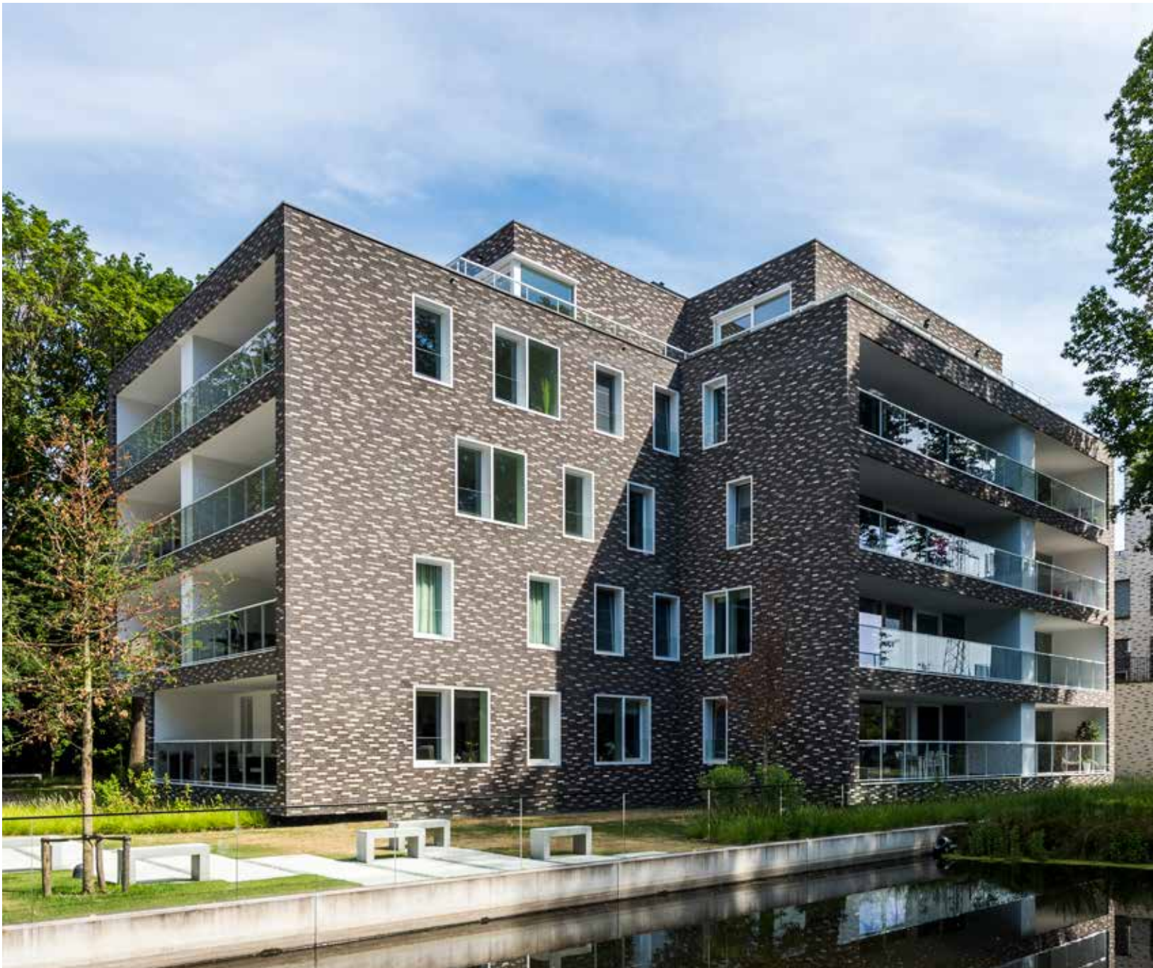
Brick mix of Terca Agora Super White, Forum Prata and Terca Patrimonia Pastorale Braised (custom-made)
