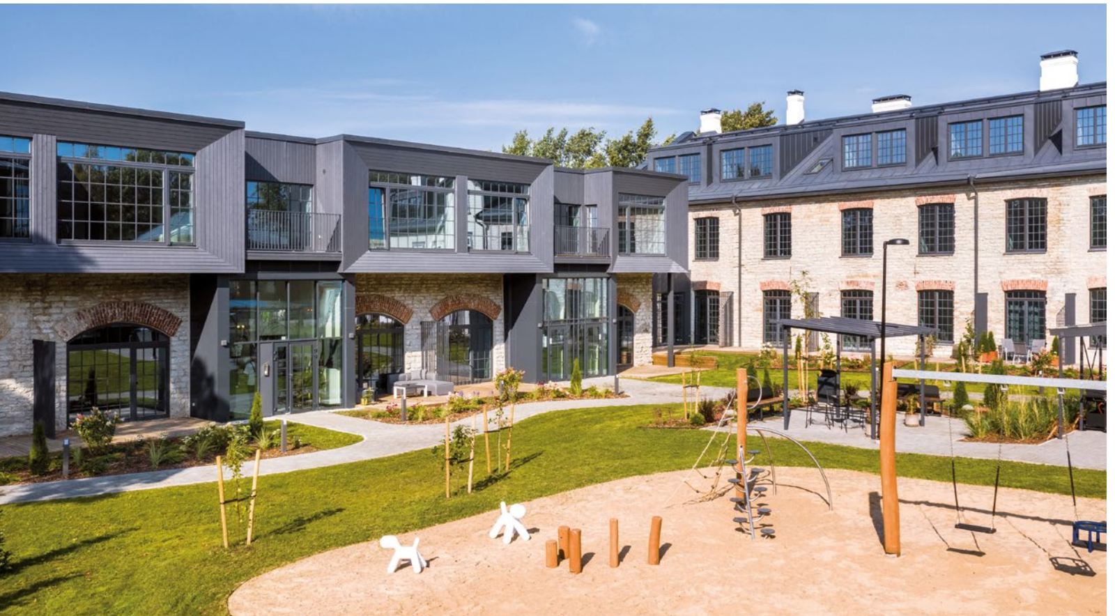
The former candy factory has been turned into a family-friendly residential complex.
