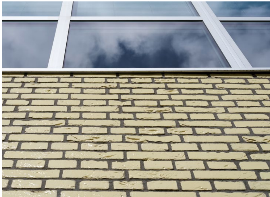
The original bricks were simple, red bricks with a pale yellow glaze applied subsequently. The new bricks are themselves yellow, but have the same texture and colour glaze as the originals.
