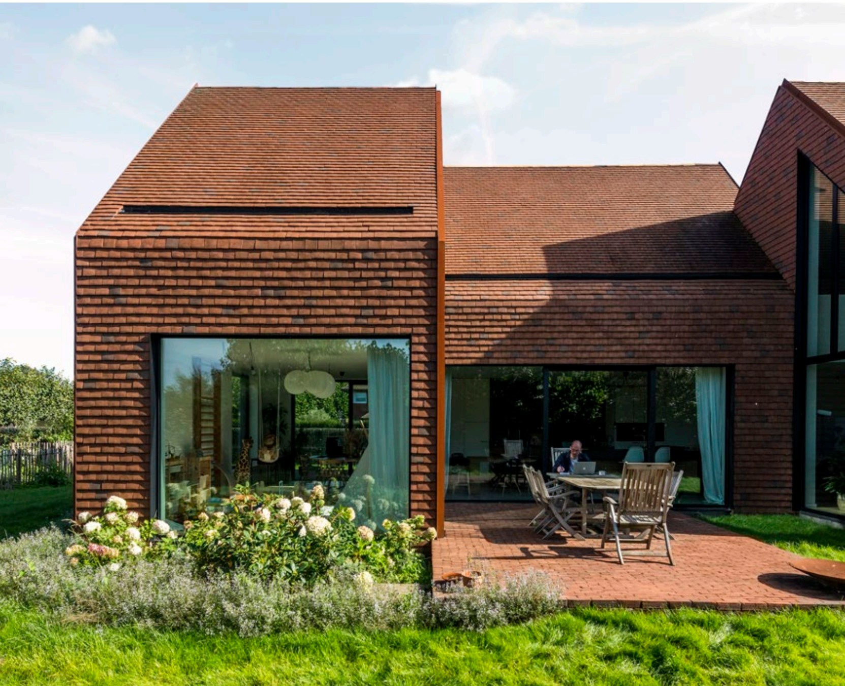
Façade and roof: tile-mix of Keymer Goxhill Autumn Brown and Keymer Goxhill Dark Chestnut. Paving: Novoton
