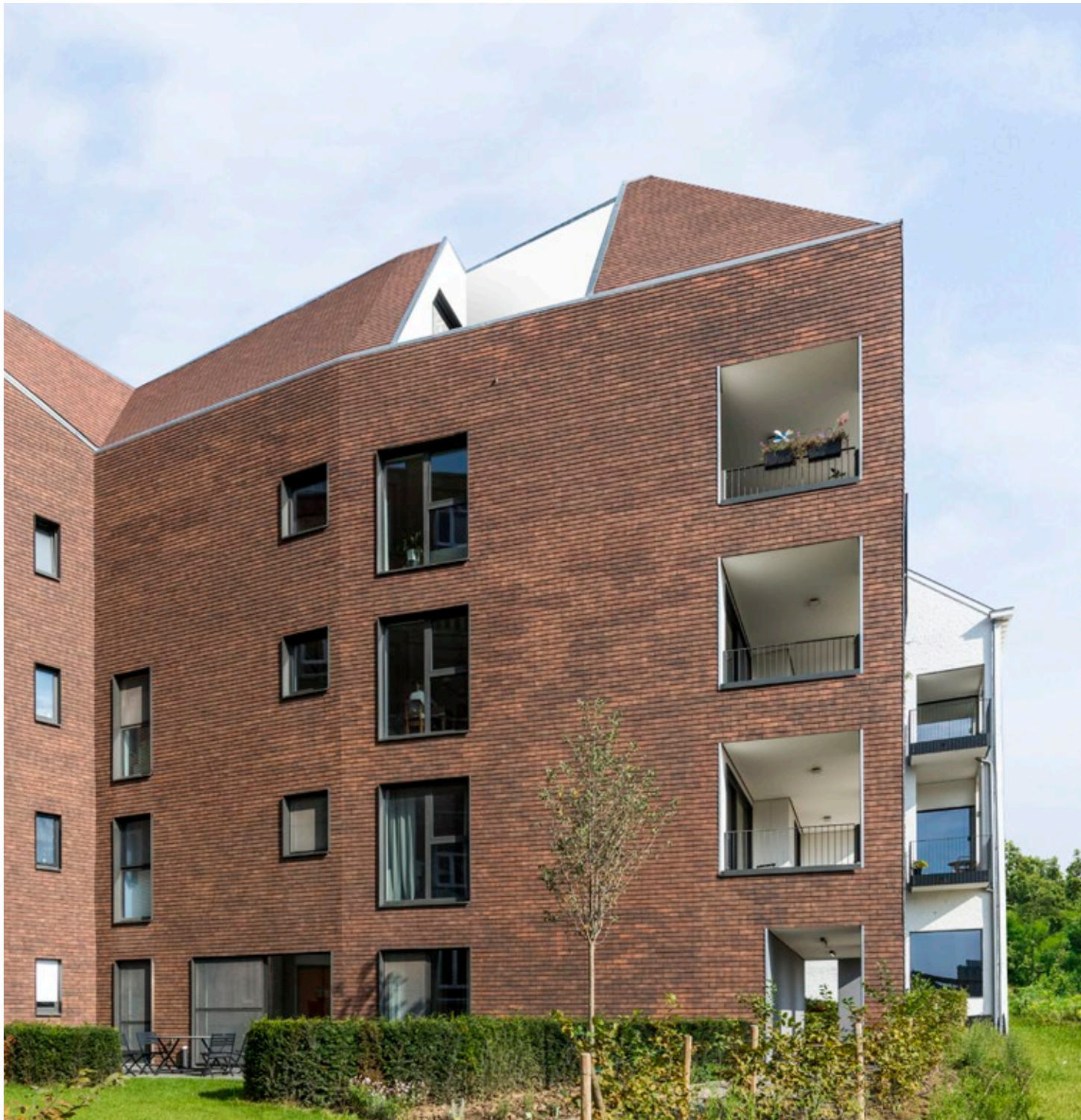
Façade and roof: Plain Tile Plato Warm Rusty Brown (custom product)
