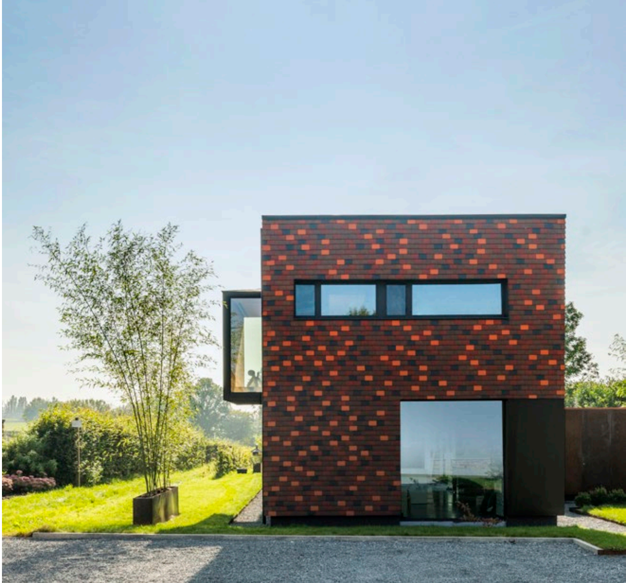
Tile-mix of Plain Tile 301 Smooth Rustic, Amarant, Braised Blue and Natural Red
