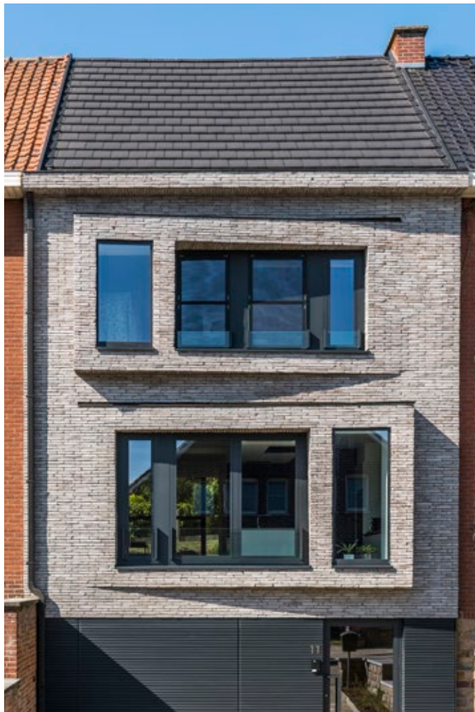
Façade: Imperium Flavius. Roof: Actua 10 Slate Engobe ZIN-architecten, Leuven
