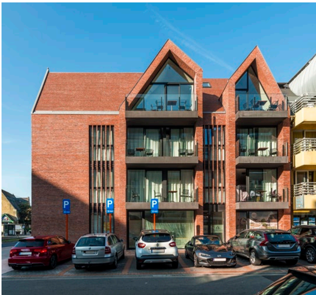
Façade: Metropolis Aula Red Eco-brick. Roof: Plain tile Aléonard Pontigny Mellow red
