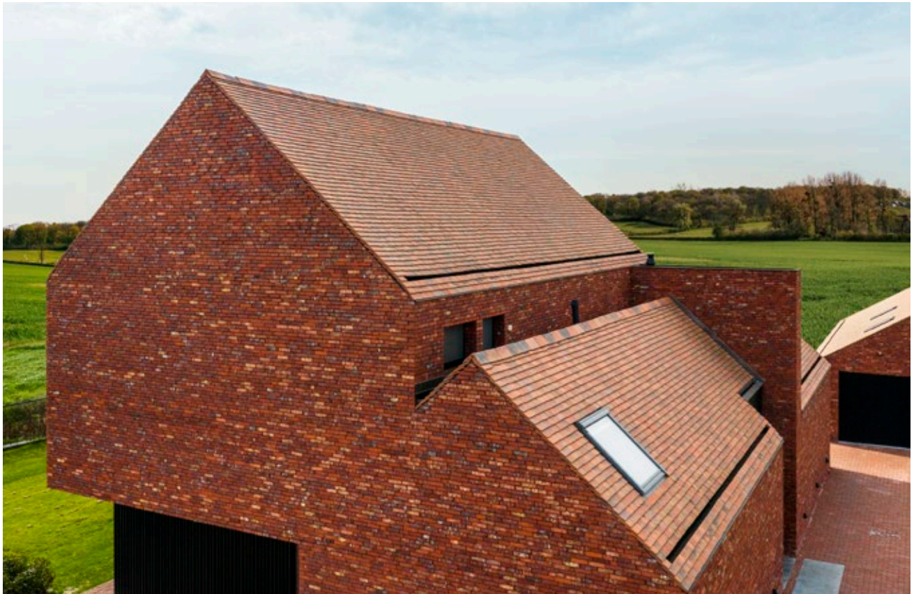
Façade: Hectic. Roof: tile-mix of Aléonard Esprit Patrimoine, Lichen Green, Kent Red and Vineyard Black
