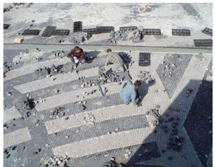
Paving layers at work in Moscow.
