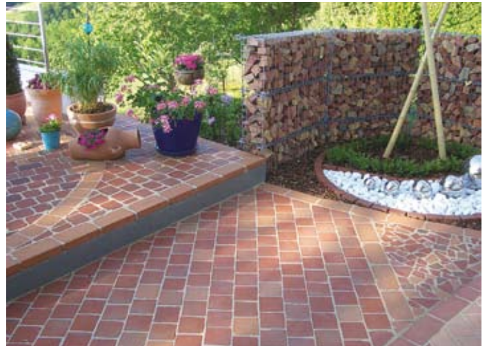
Original design: Broken pavers were tipped into a gabion.
