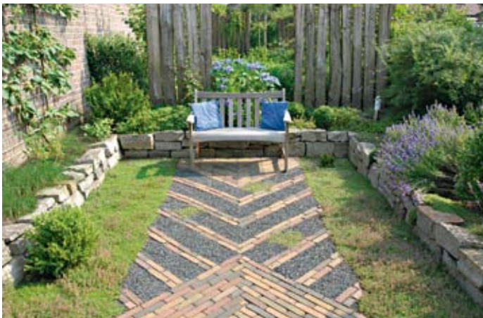
An oasis for the aesthete on just 80 square metres: paths of Dutch pavers laid flat and on end and gravel lead through the garden.
