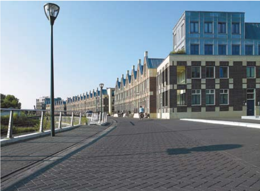
IJsselkade, Doesburg: The typical red colouring of the paving bricks creates the link between contemporary housing development and the cultural and historical appearance of the characteristic old town buildings. Paving bricks used: Nero DF and KK70 deep black
