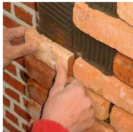
Our on-line pressed brick slips are available with a thickness starting from 9mm.
