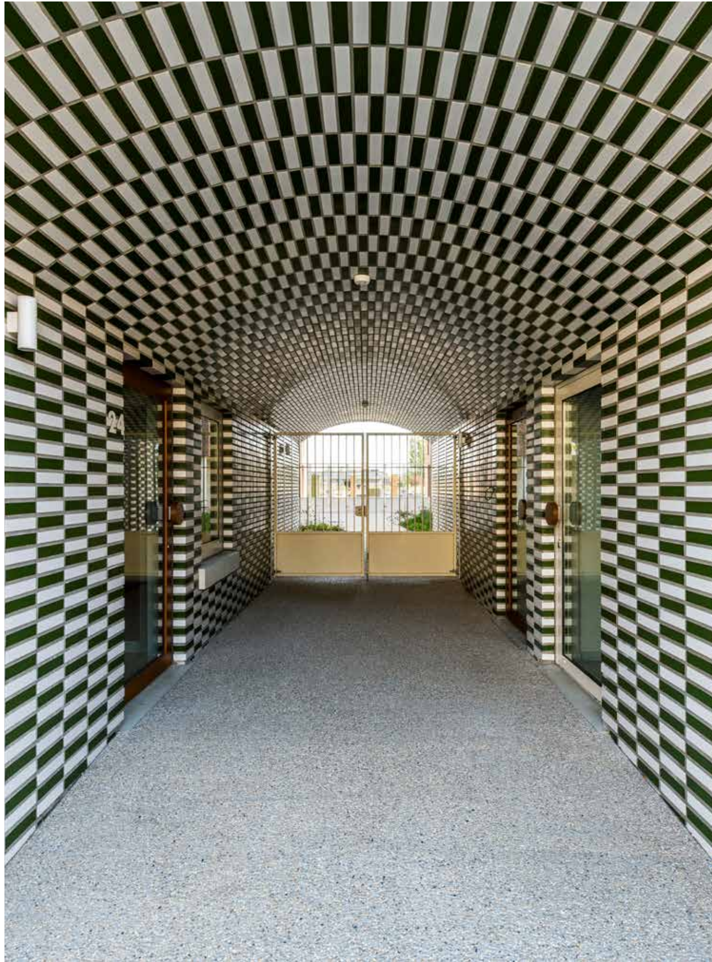
Mix of glazed bricks
