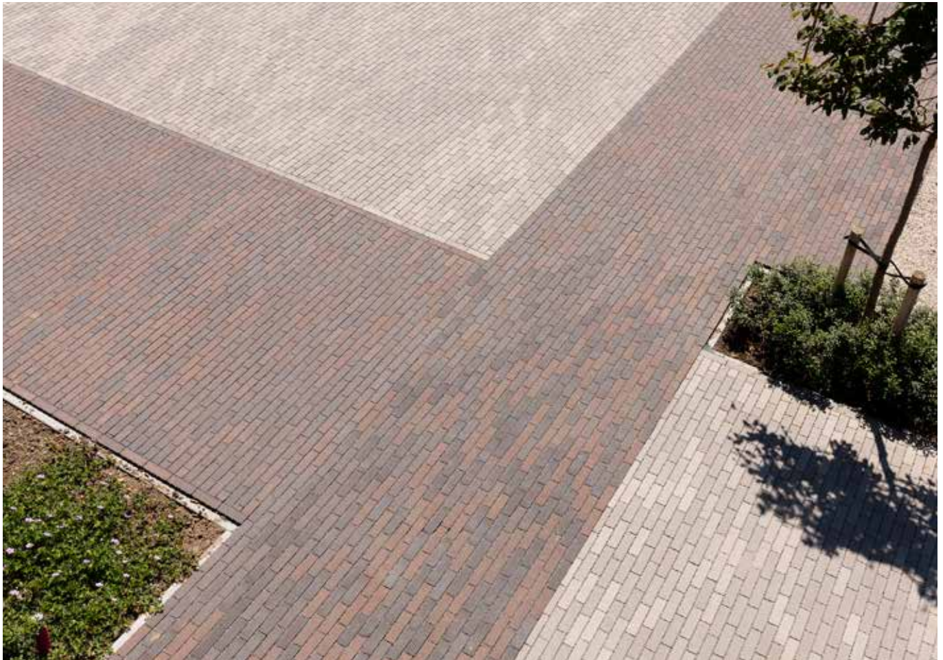
AQUATA BROWN Dudzele Village Centre, Belgium
